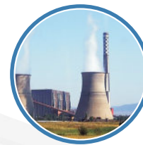
Energy Plant Entrances
