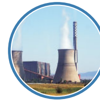
Energy Plant Entrances
