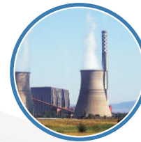
Energy Plant Entrances
